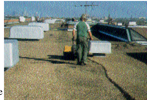
Remove loose gravel and clean roof system prior to installation.
